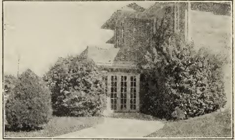
Evergreens Growing Around Porte Cochere
